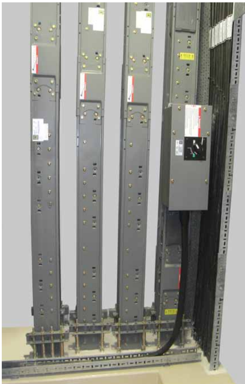
Typical busbar riser system including plug-in circuit breaker
